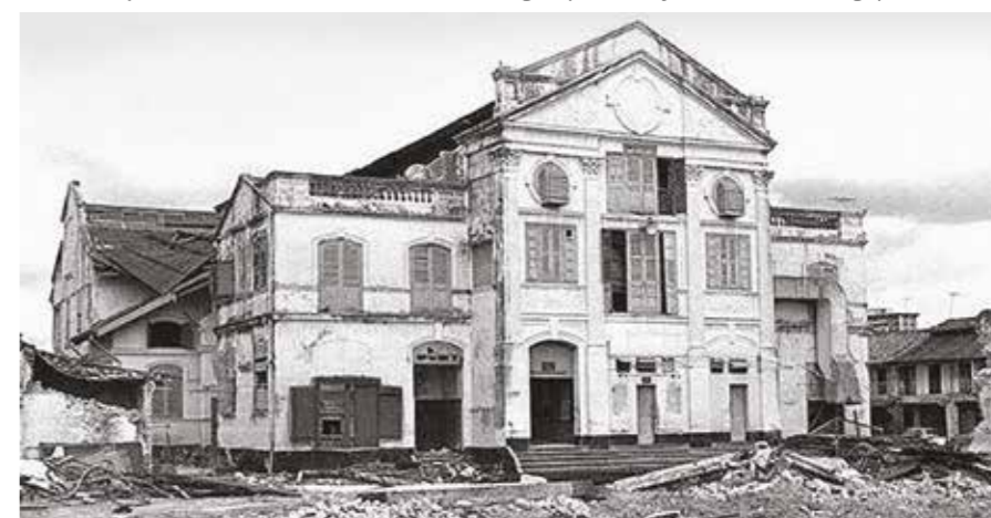
Theatre Royal in the midst of demolition in 1977. Image reproduced from Remember Singapore website.
